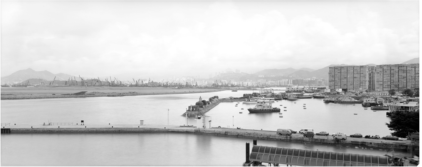
Lois Conner, Kai Tak airport construction, Hong Kong, 1993 Platinum print, 6 1/2 x 16 1/2 in. (16.5 x 41.9 cm) 5888
